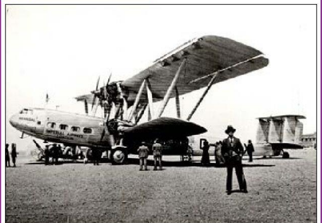
This historic picture of a Handley Page 42 aircraft at Bahrain Airport was taken in the early 1930s
